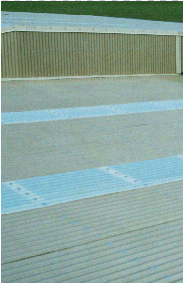
Pivot PFC Warehouse, Keith, S.A.
